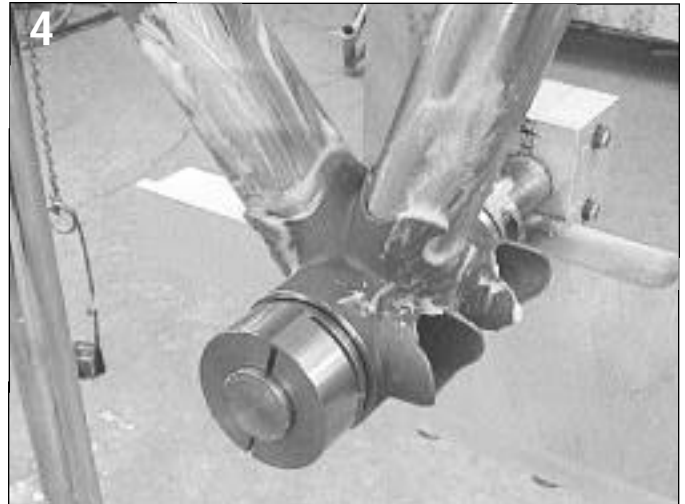
4 Here's the BB fluxed and assembled in the frame fixture, where it is tacked. I take it out of the fixture for brazing.
