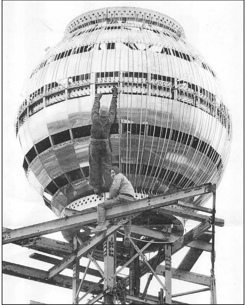
Ian cuts the wires on the Channel 13 Weatherball, on the way to a full restoration. The 15' diameter stainless steel ball mounted on a 120' pole in Grand Rapids is overlaid with 2880' of neon. A new one built today would run somewhere around $200,000.
